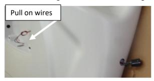
8. Remove defective wires with a regular slotted screwdriver and connect the new one to the junction box.
